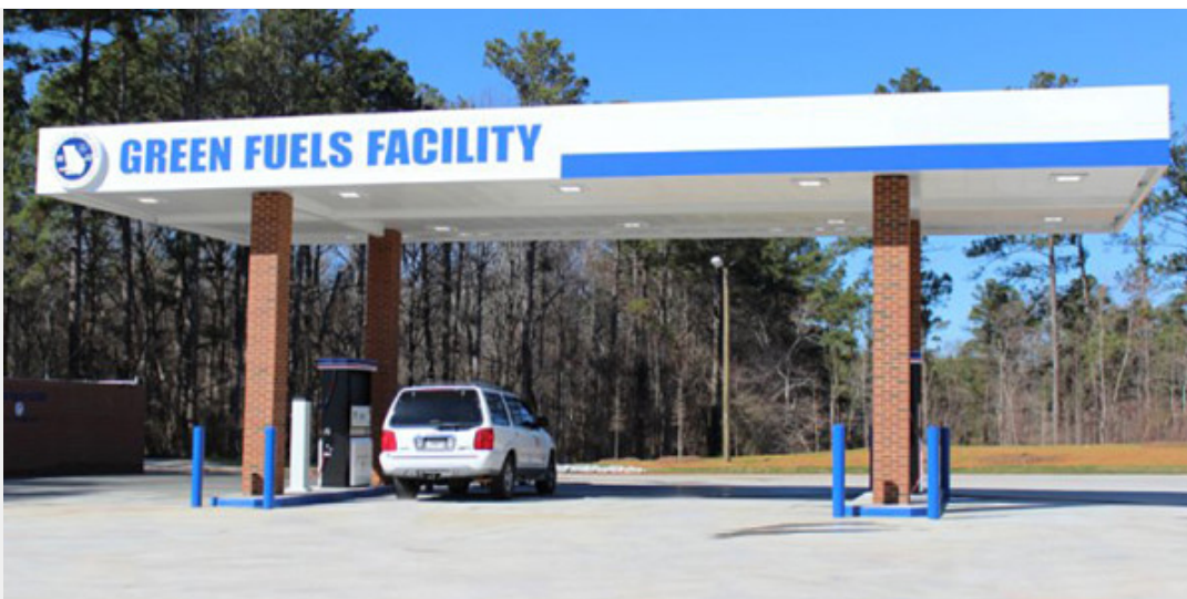
$1.6 million facility by American Fueling Systems in Covington is the first public access CNG station in Georgia to be owned by a city, AFS says.
